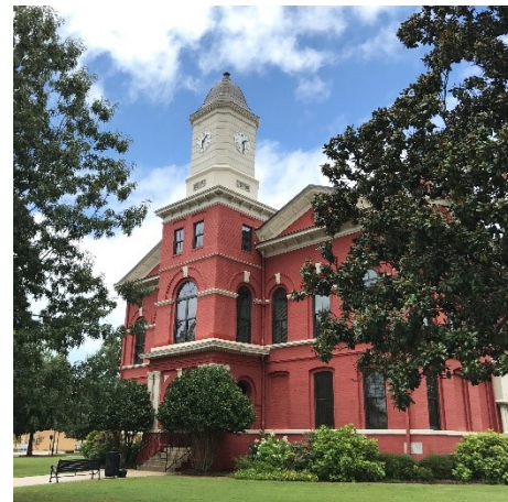
Figure 2: Pike County Courthouse in Downtown Zebulon
