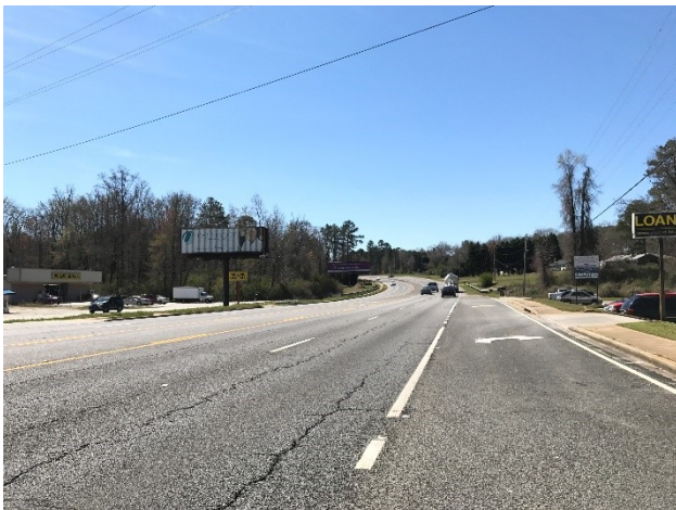
Figure 15: Highway 19 in south Zebulon
